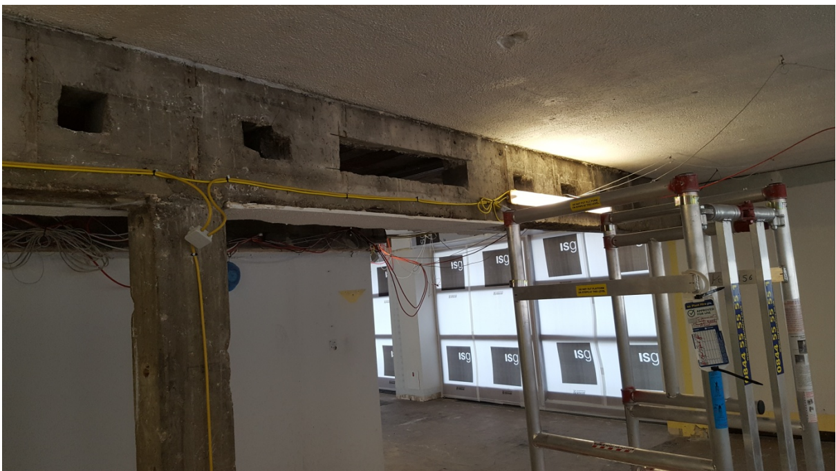
Plate 4 – View onto service holes in down stand beam (2)
