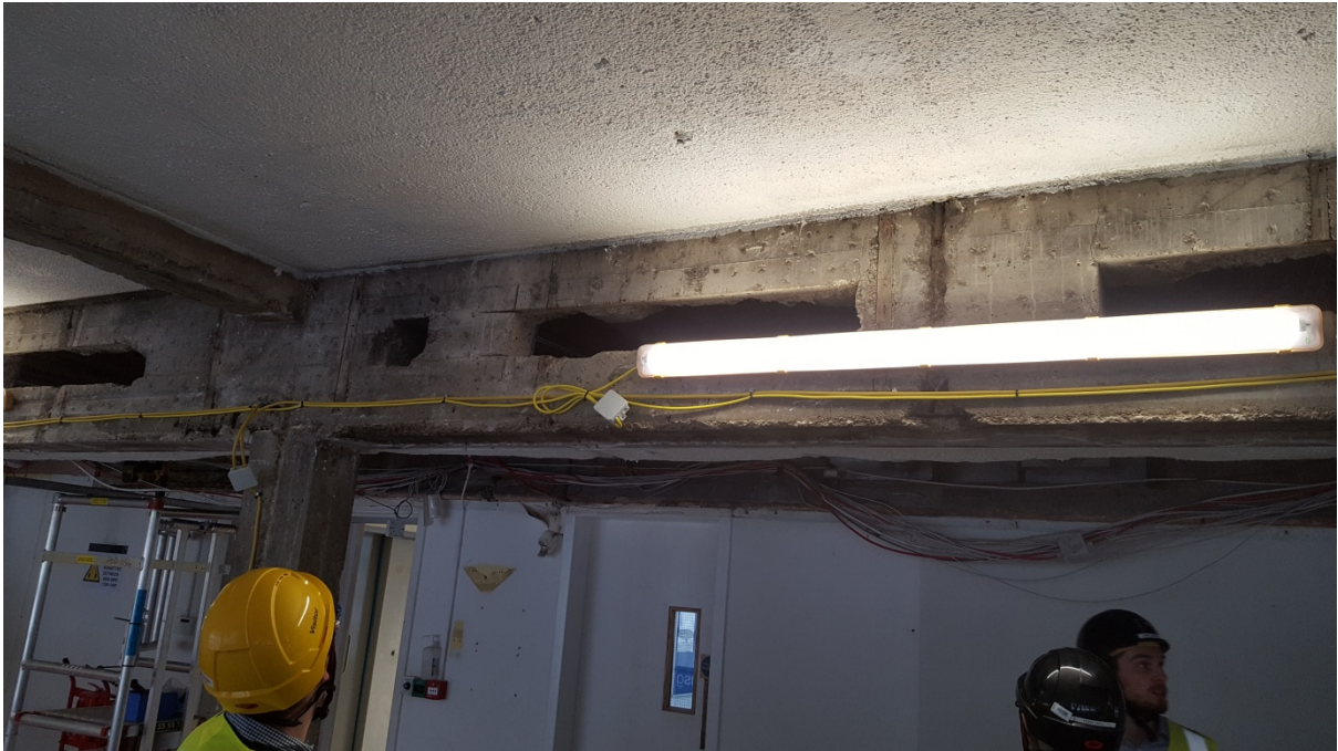
Plate 3 – View onto service holes in down stand beam (1)
