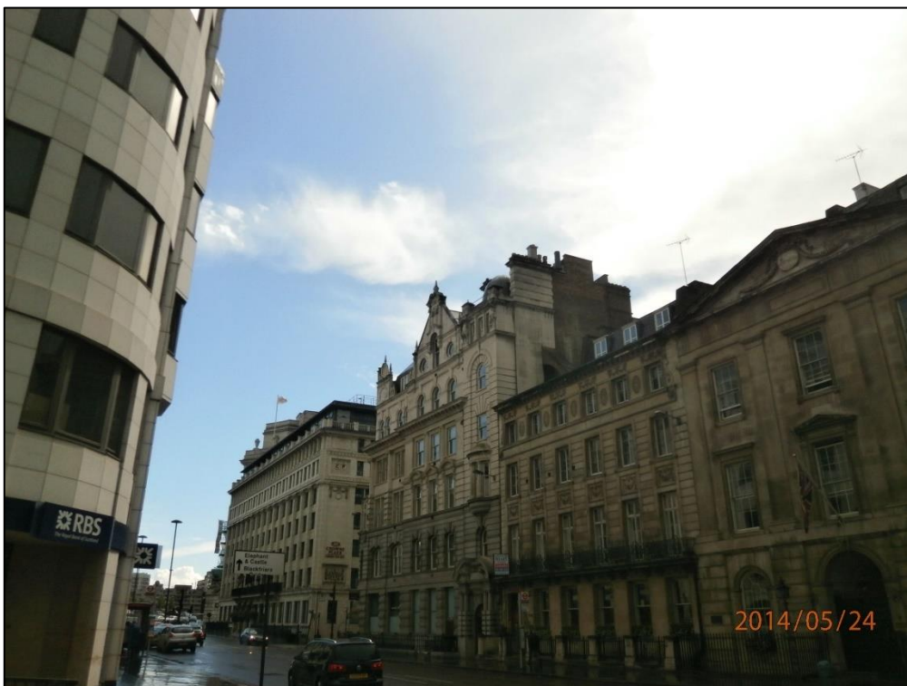
Figure 2b: GRP chimney from Figure 2a, from street level
