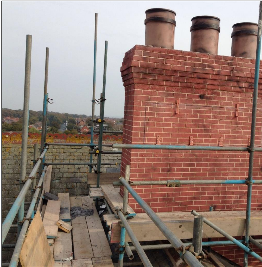
Figure 2c: GRP chimney very close up, with GRP chimney pots
