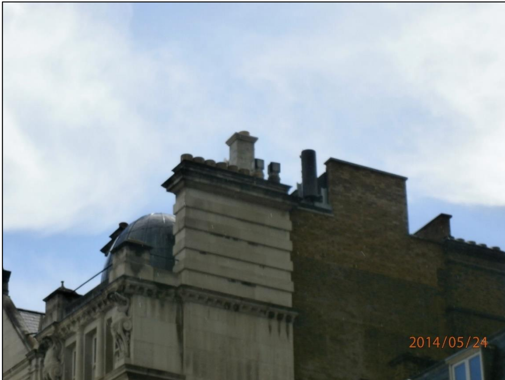
Figure 2a: GRP chimney close up
