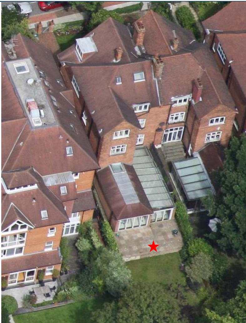
Figure 2: Birdseye View from south
