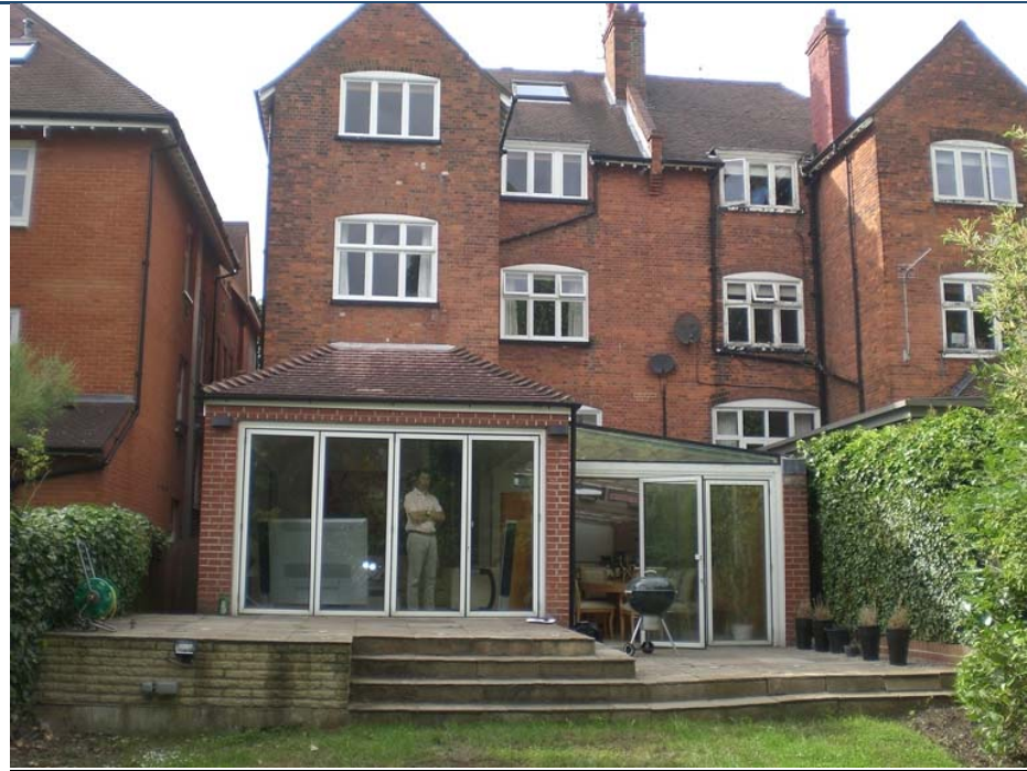
Figure 13: Rear elevation of existing property
