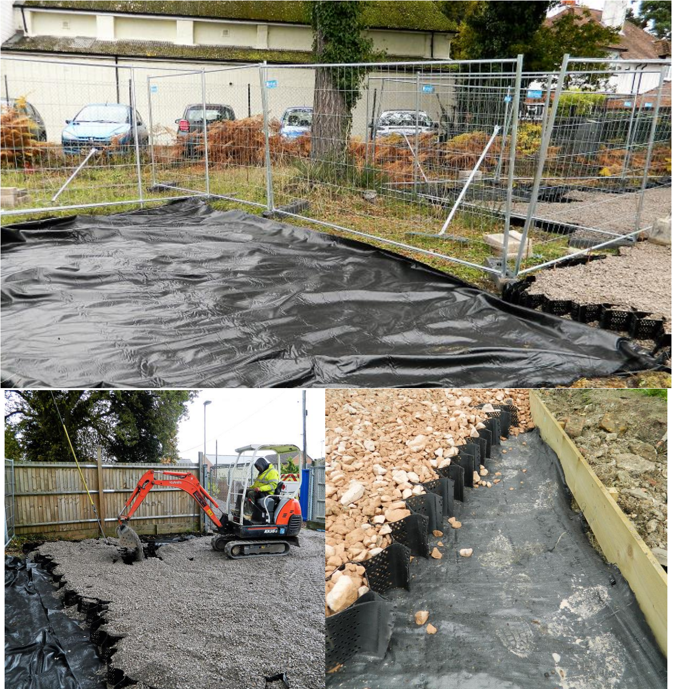
Figure 8. Photographs illustrating cellular confinement system used to form an above-ground no-dig driveway
