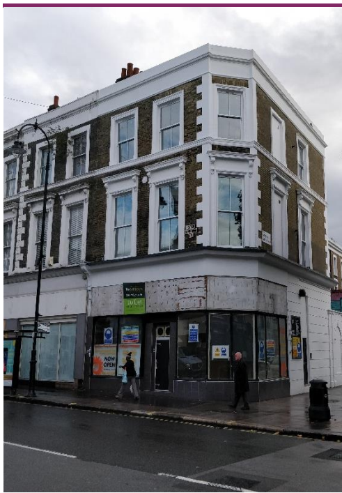
F.2 Existing Shopfront
