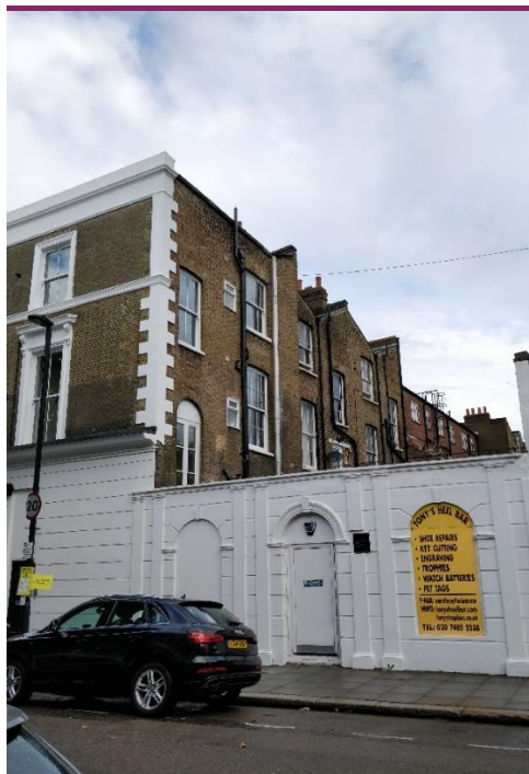
F.3 In-filled Windows along Gaisford Street
