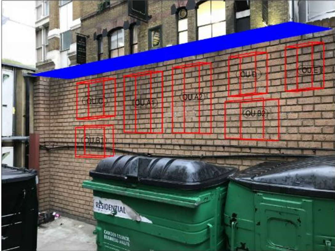
Figure 3 – Proposed arrangement of new plant (red) and acoustic roof/lid (blue)
