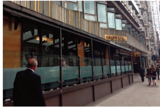
The Imperial Hotel, External Seating Area
