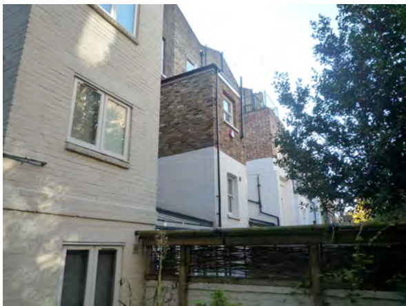
Photograph of existing rear outrigger, looking west
