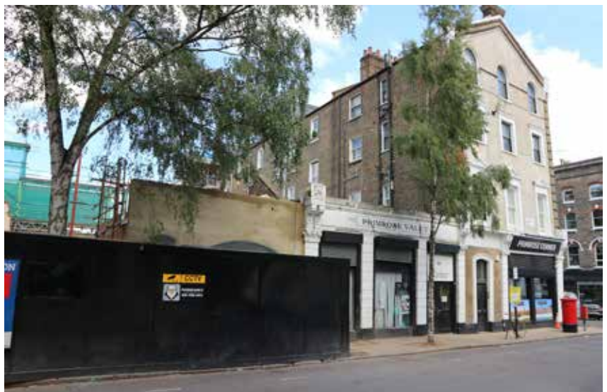
38 View of rear of 91-99 Regent's Park Road, from Erskine Road.
