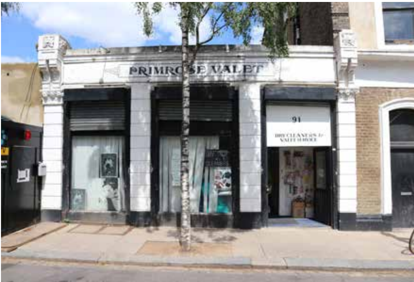
41. Front elevation of No.91a Regent's Park Road.
