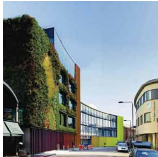
2. Existing view from Hawley Crescent towards the east
