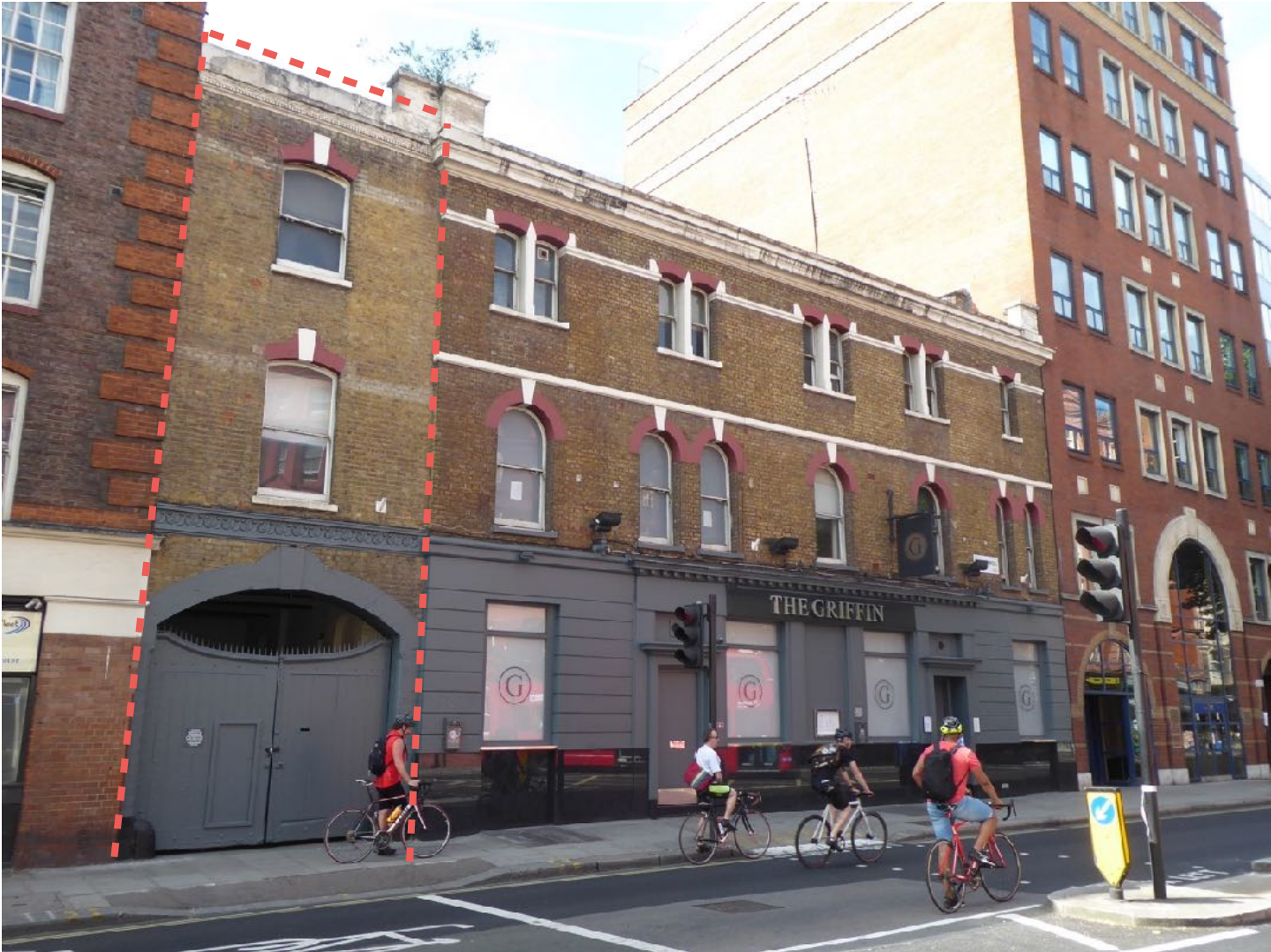
Front facade of 125 Clerkenwell Road. The proposed section of the facade to be demolished and then re-built is the eastern-most section of the elevation (within red dotted line) which is set back by half a brick.
