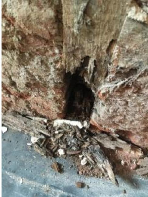
***Photo 1 – Example of rotten embedded timbers***
