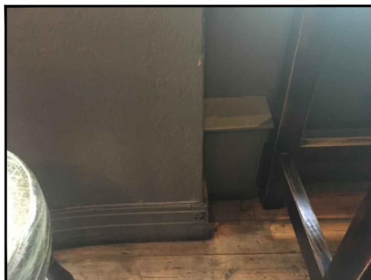
EXISTING GROUND LEVEL RISER BOXING FROM BASEMENT
