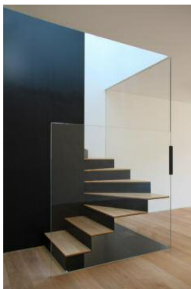
STEEL / TIMBER / GLASS STAIRCASE BETWEEN GROUND FLOOR AND LOWER GROUND FLOOR
