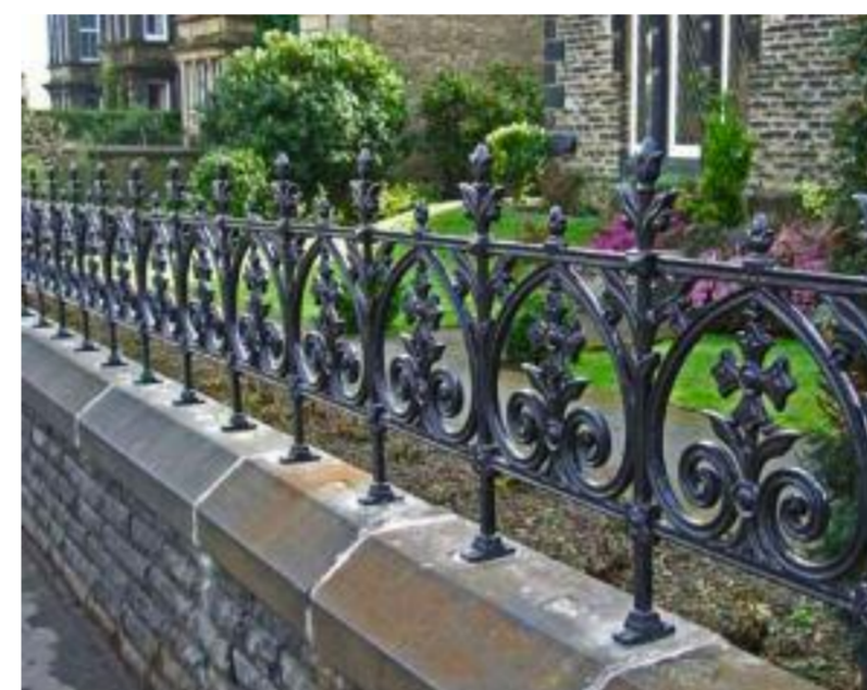
EXTERNAL BALUSTRADE: REPRODUCTION EDWARDIAN CAST IRON RAILINGS - PAINTED
