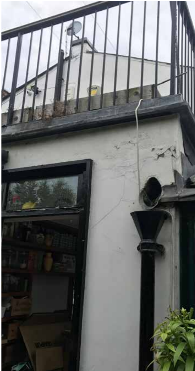
Existing roof terrace, balustrade and rear wall
