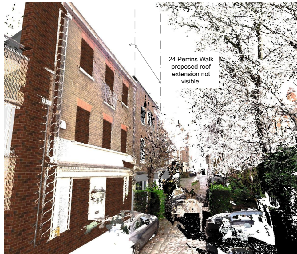
View from bottom of the street combined with point cloud
