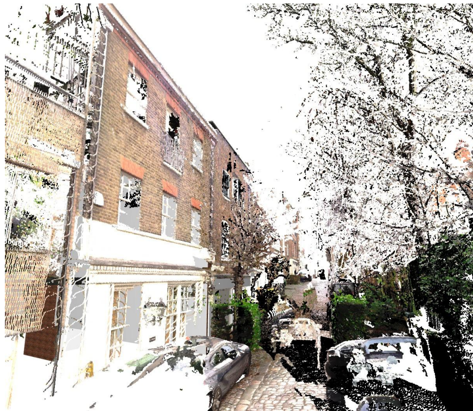
View from bottom of the street -PC
