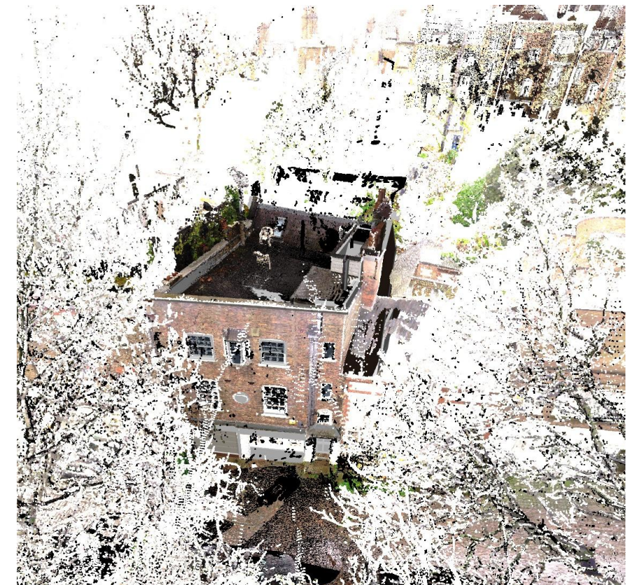
view- top roof - PC
