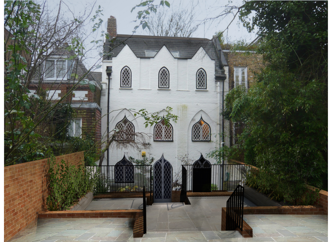
Revision E Proposed rear view from rear of garden including mansard roof over new roof extension
