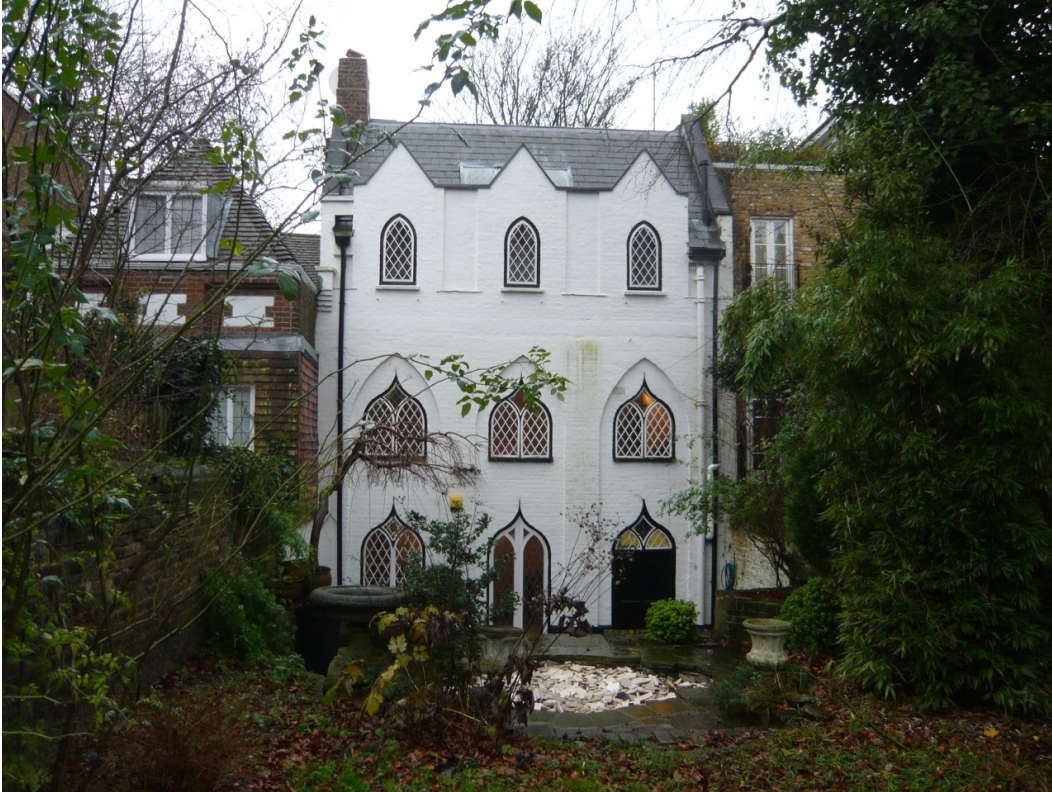
Existing rear view from rear of grade without proposed roof extension.
