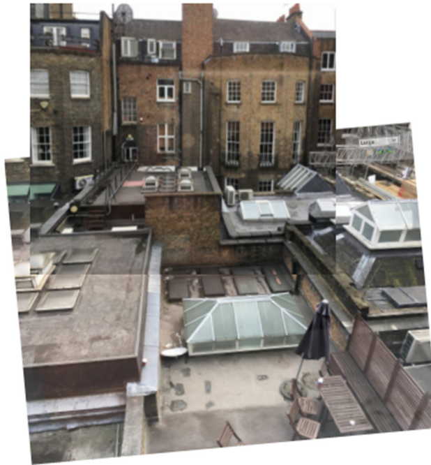
Existing roof scape viewed from the rear of 4 Windmill Street
