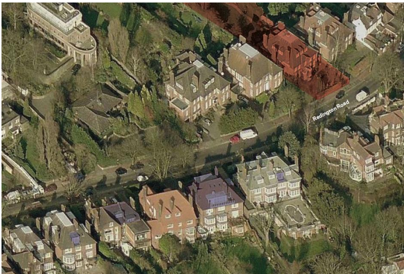
Aerial view showing a sample of other roof terraces in the immediate context
