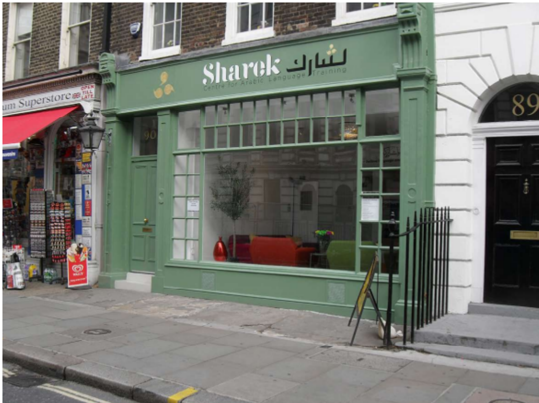
Photo 3 – shopfront elevation (existing view)
