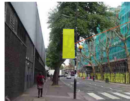
EVERSHOLT ST. / PHOENIX RD JUNCTION
