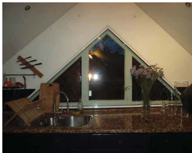
Existing window WGF-12
