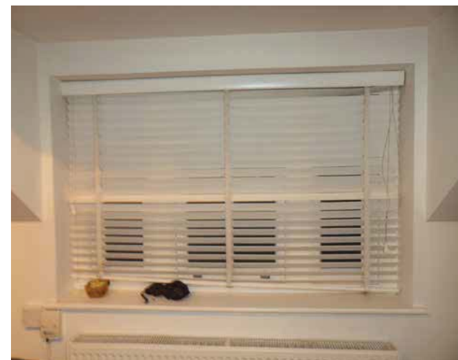
Existing window WGF-11
