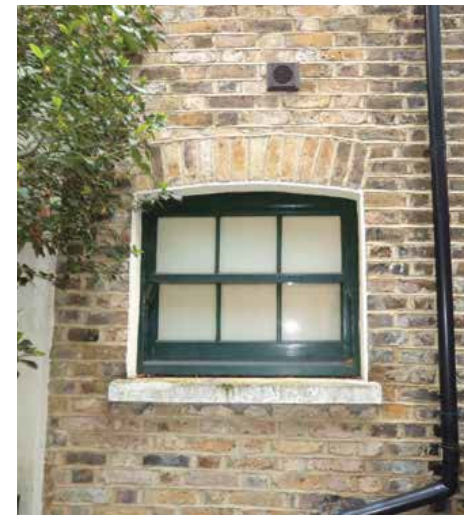
Repairs to brickwork
