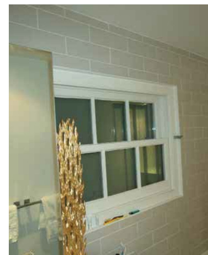
Internal view of existing window WLGF-10
