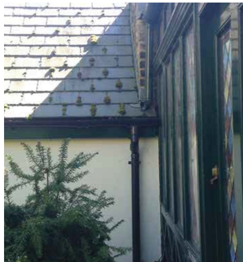
Repairs/rationalising rainwater goods
