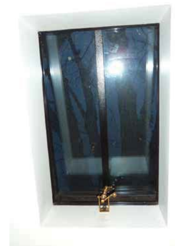
Existing roof light WRL-02
