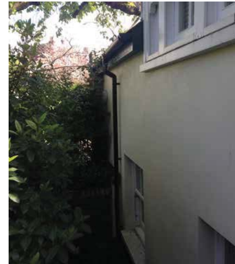
Repairs to gutters
