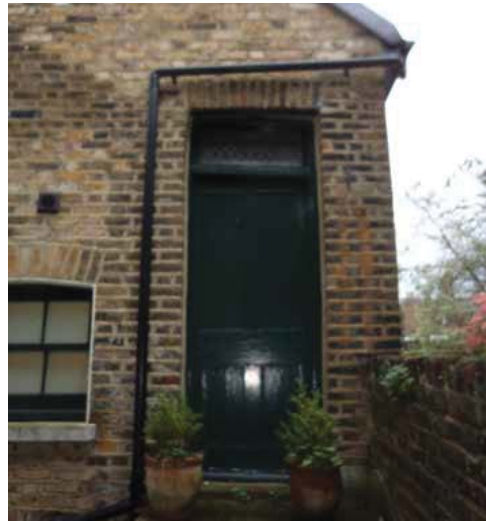
Repairs/rationalising rainwater goods
