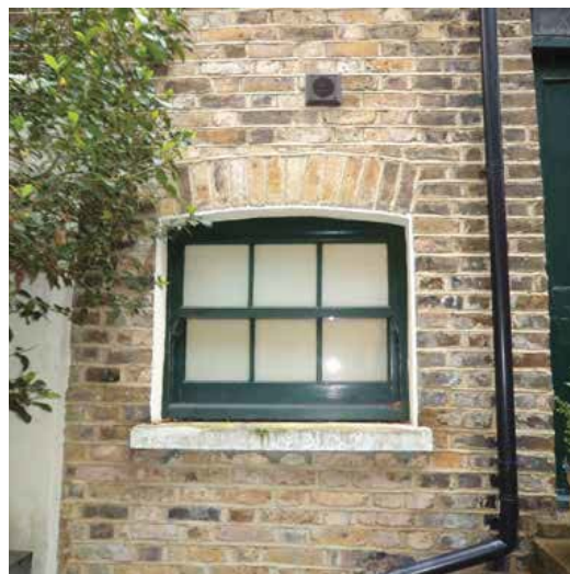
External view of existing window WLGF-10
