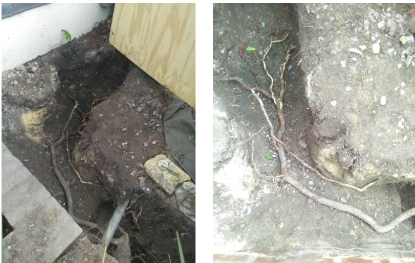
C: Photograph of trial trench extending to south of existing lightwell where 1 x minor root exists
