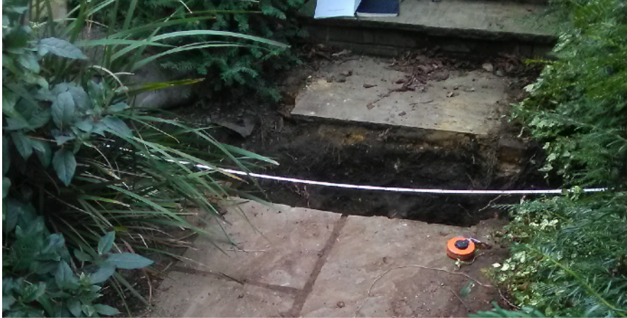
B: Overview photographs of trial trench as viewed from above and within pit
