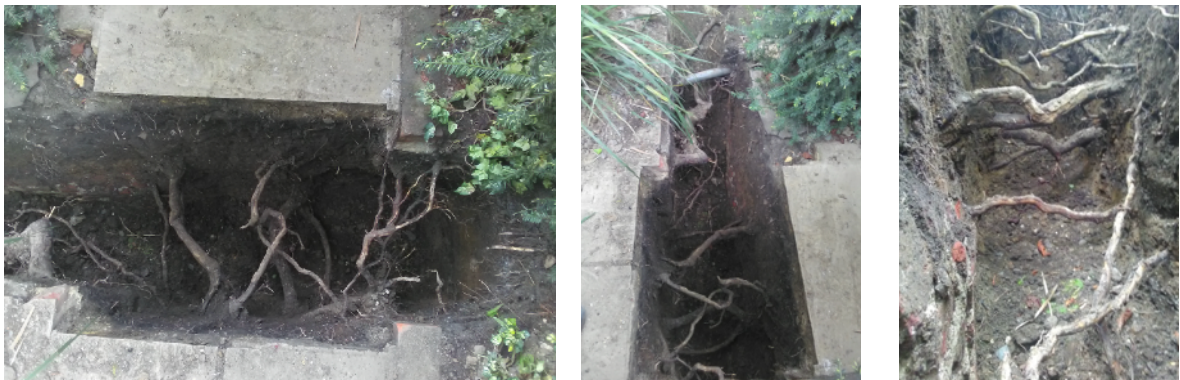
C: Photograph of trial trench extending to south of existing lightwell where 1 x minor root exists
