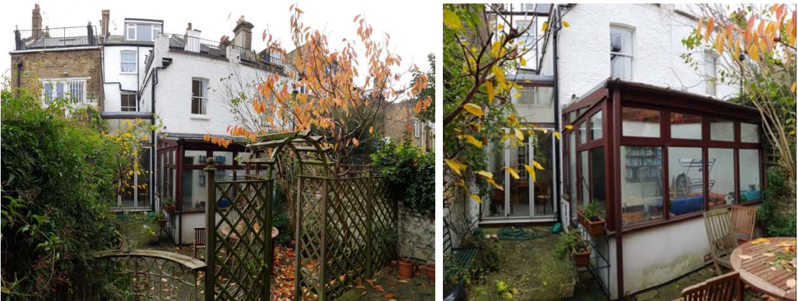
Rear views of the property
