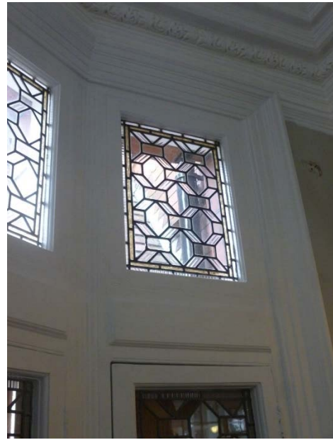
Head rail to be fitted on transom. Raised panels to be retained and protected.
