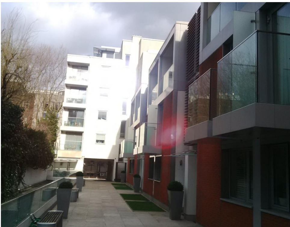
Crabtree Place town houses and flats
