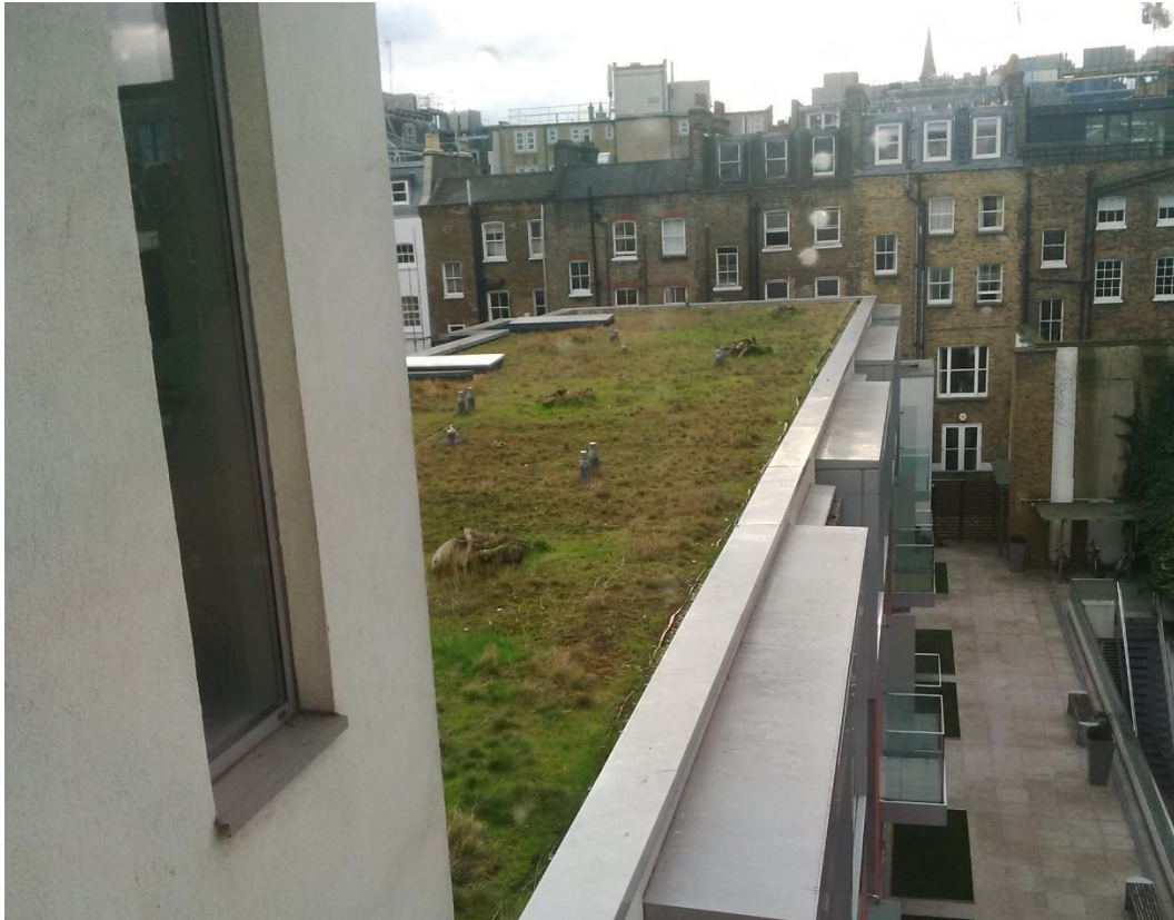
Crabtree Place existing green roof
