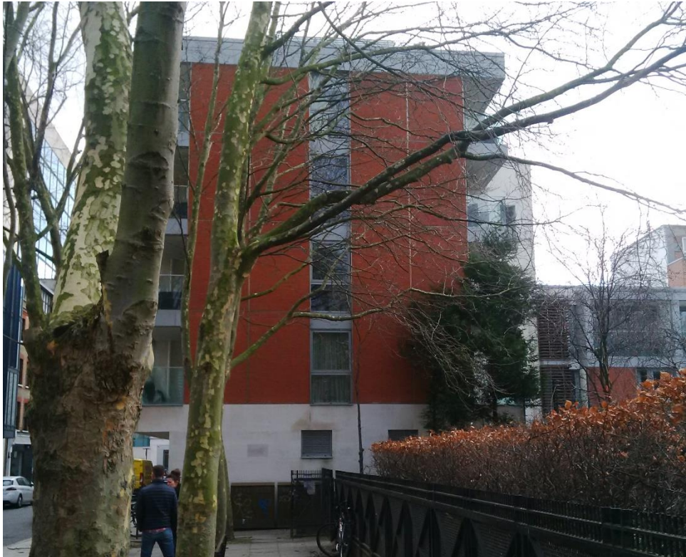
Crabtree House / Place - 6 storey front element
