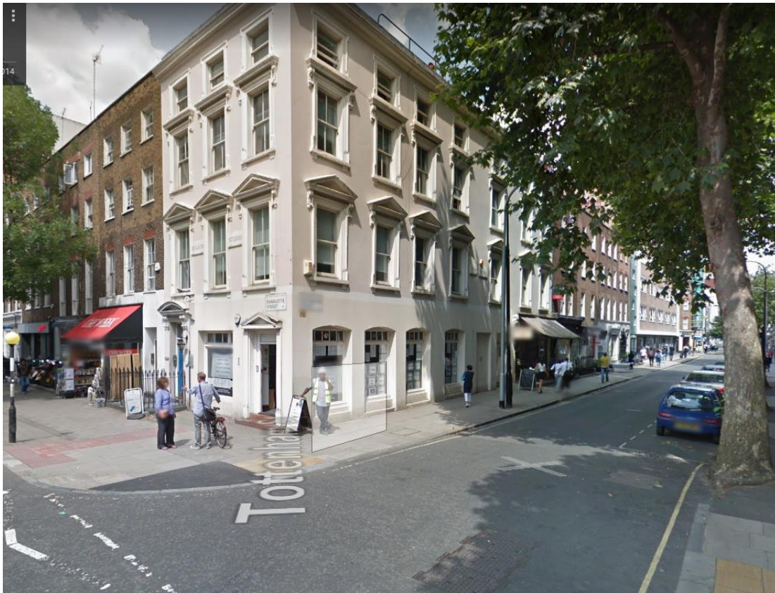
Photo 3 - Pre-existing photo of the flank elevation of 64 Charlotte Street also showing 32 Tottenham Street
