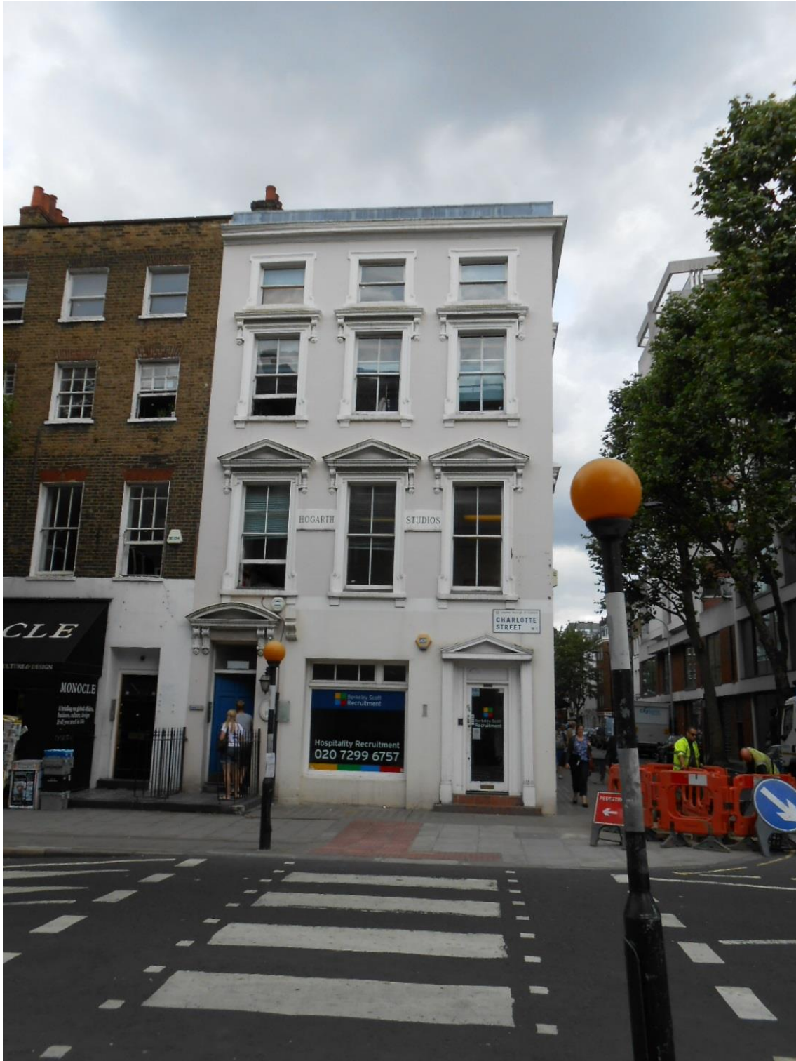
Photo 2 - Pre-existing photo 64 Charlotte Street
