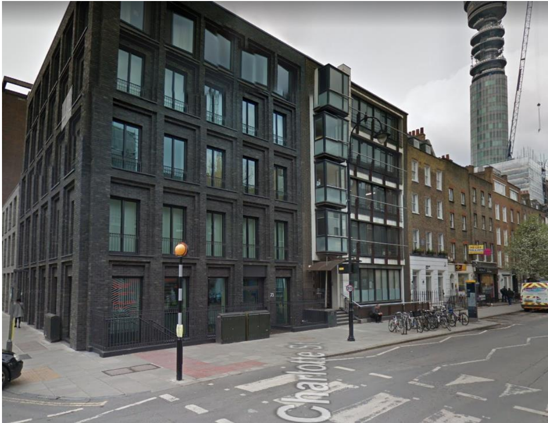
Photo 5 - Photo showing the properties opposite the site at 73-79 Charlotte Street
