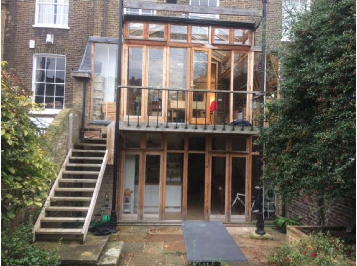
Photo 2 - Existing two storey conservatory extension at 13 Gloucester Crescent
