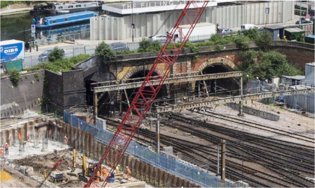
Fig. 2 - Gasworks Tunnels & 'Box Abutment'
