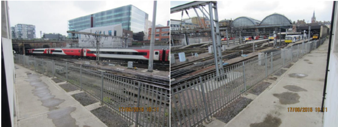
Fig. 4 - Tracks and Overhead Line Equipment (OHLE)
