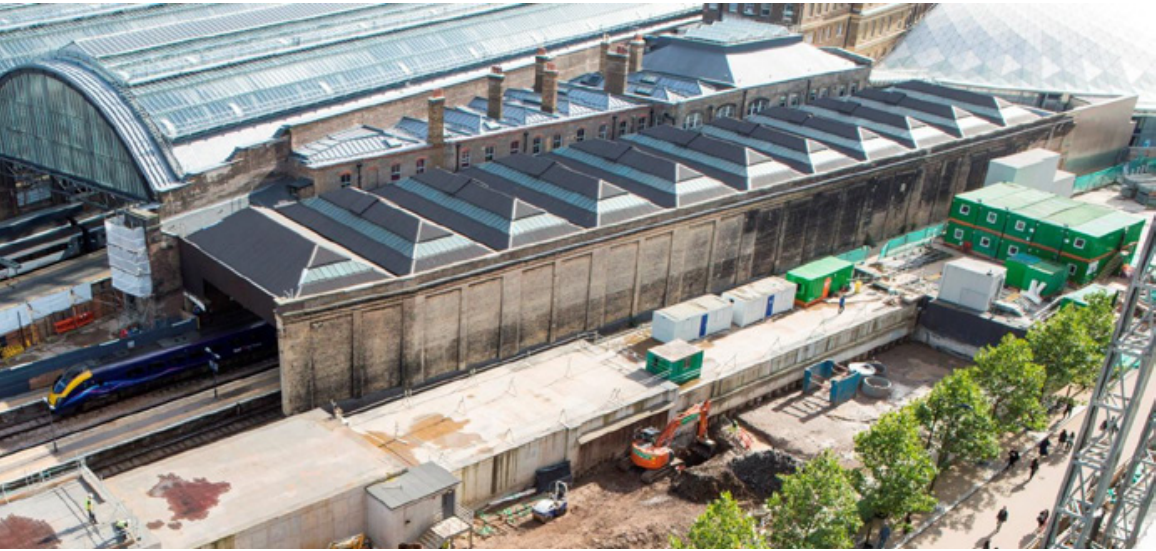
Fig. 1 - Photo of the Suburban Train Shed
