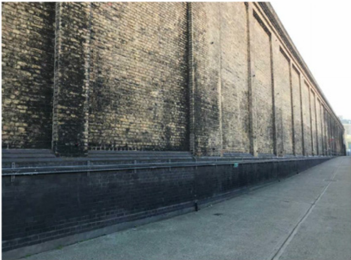
External access route
