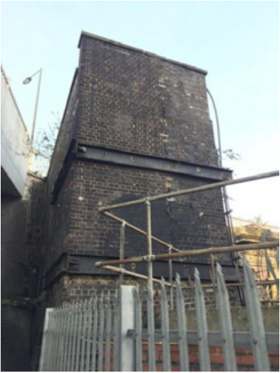
Fig. 3 - Close-up of the 'Box Abutment'
