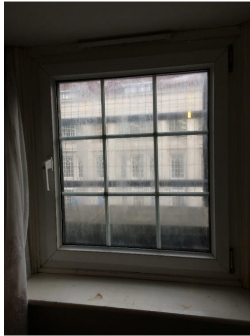
Above: PVCu TiltTurn window on dormer extension
