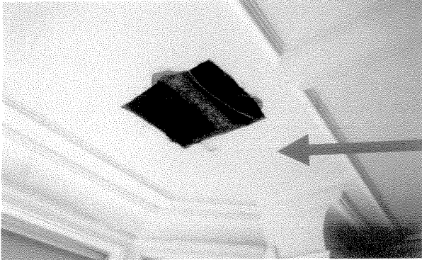
Location Ref 3: Visual Inspection- Master Bedroom - NO ASBESTOS DETECTED.
