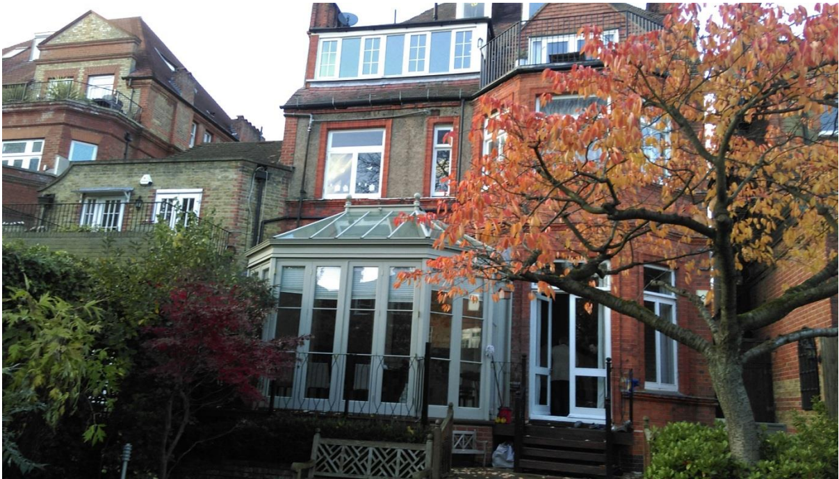
Existing rear elevation showing the conservatory (to be replaced)
