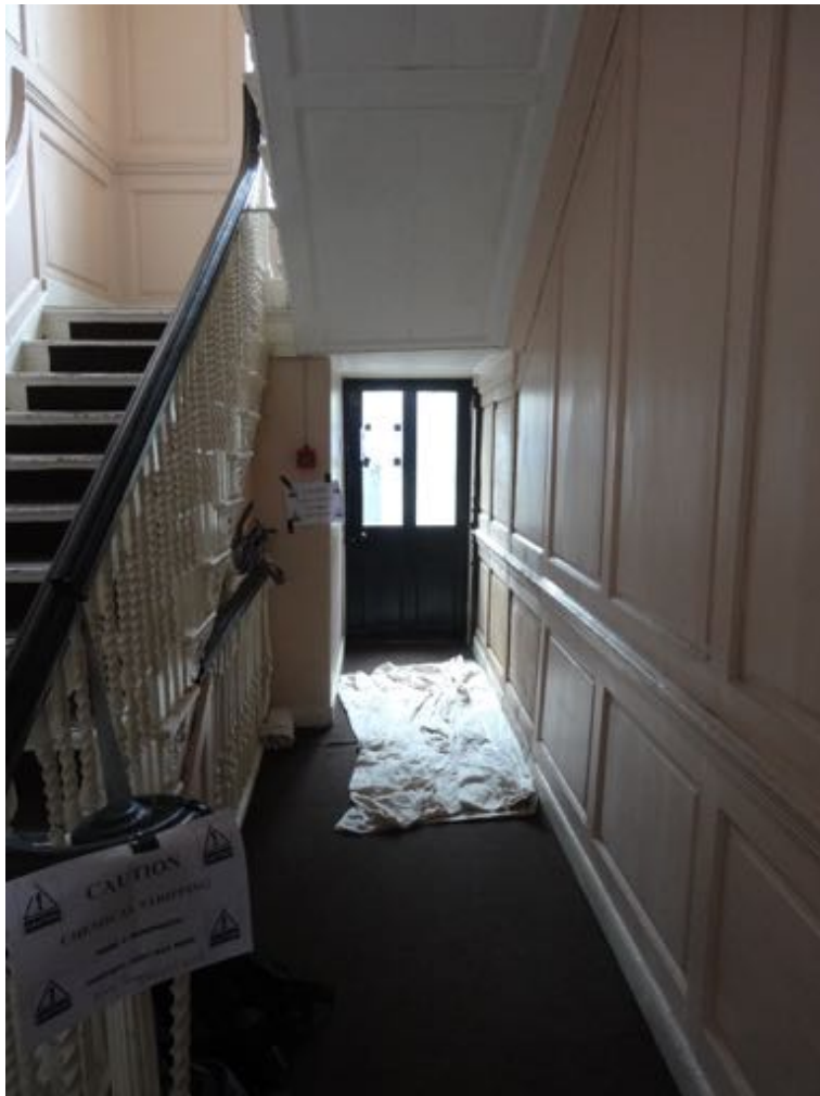
Figure 2: View of the ground floor corridor looking north, showing original panelling on the walls and the staircase with carved balusters and tread ends, March 2017.
