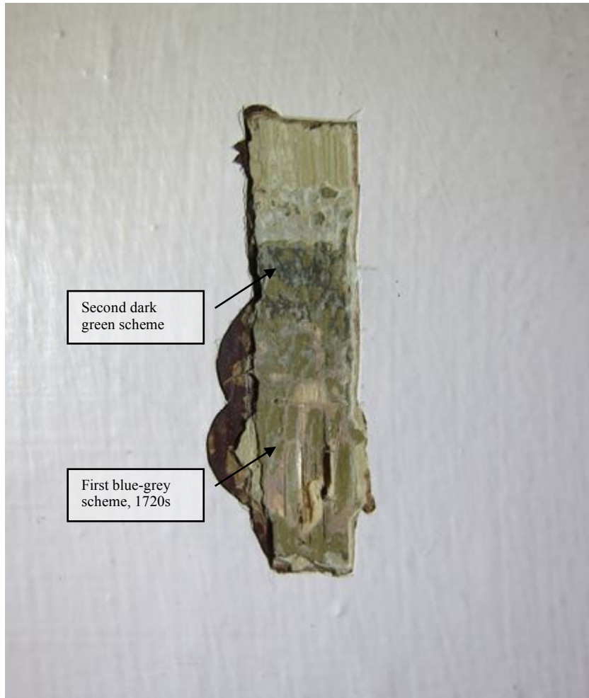
Figure 5: Uncovering showing the first, light grey-blue scheme at bottom (much of which is discoloured to a yellowish-green), fragments of the second dark green scheme at centre, and later paint schemes at the top. Uncovering ~10mm wide.
