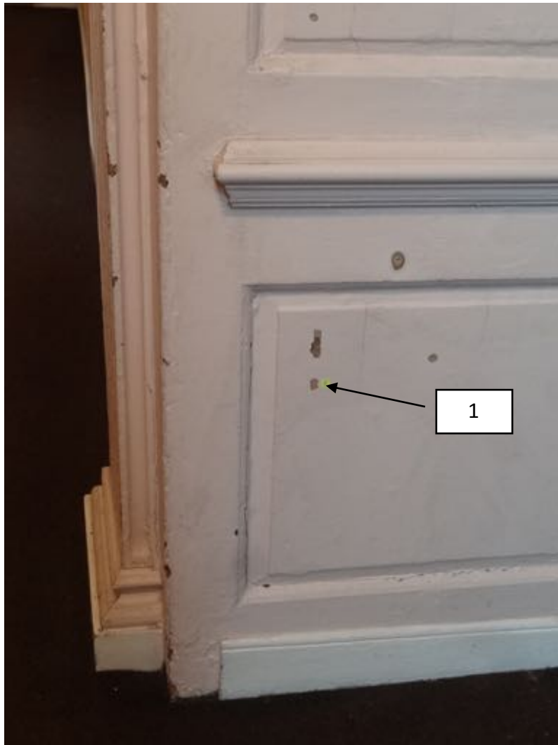
Figure 21: Location of Sample 1 on west wall panelling
