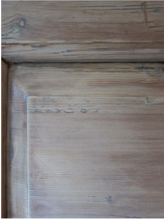
Detail of the timber surface after paint removal
