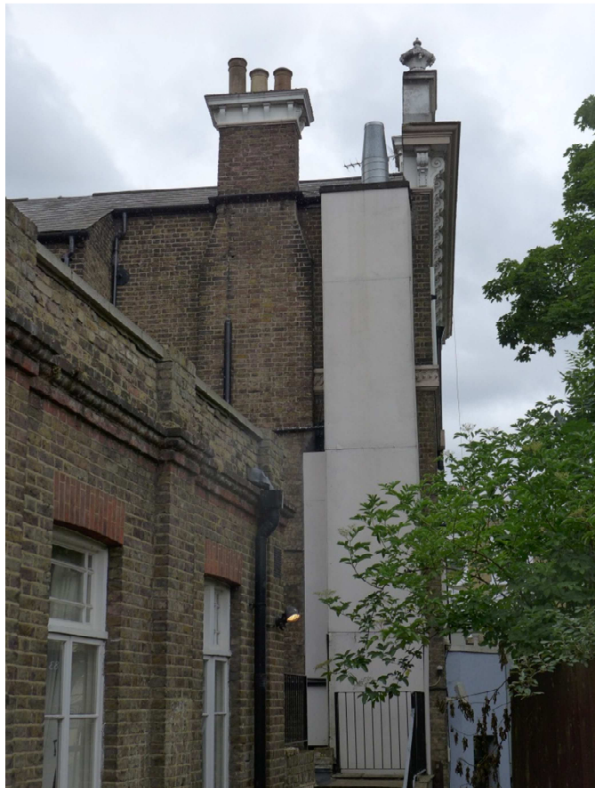
Rear elevation with service riser enclosure (white/grey colour)
