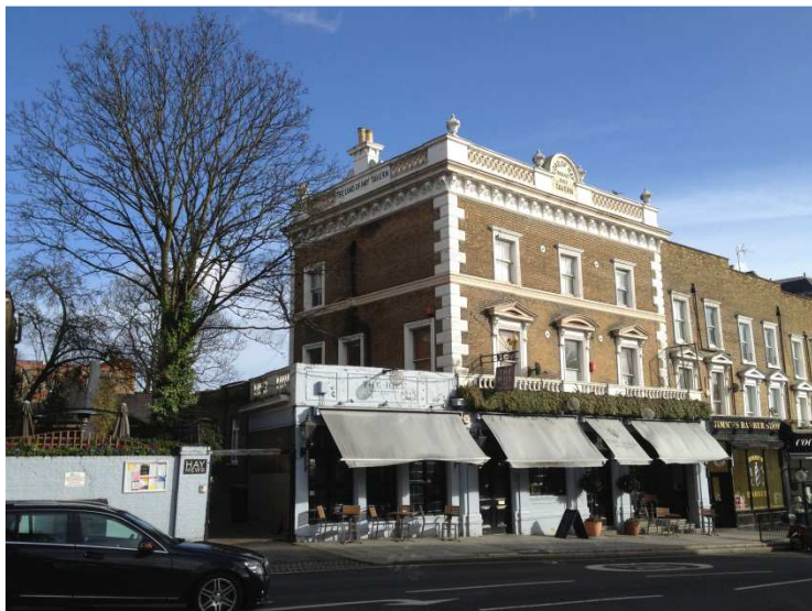
Street view of the existing building (prior to mansard extension)
