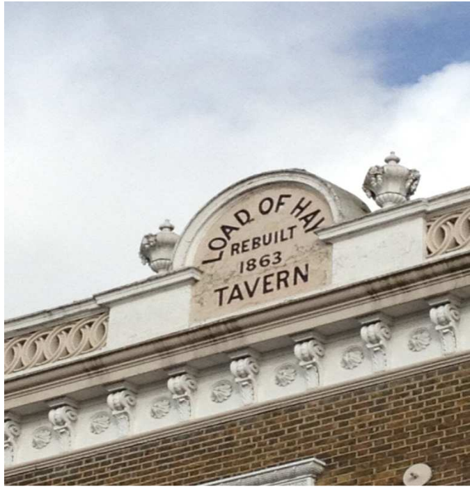
Hays Mews front parapet decorative detailing
