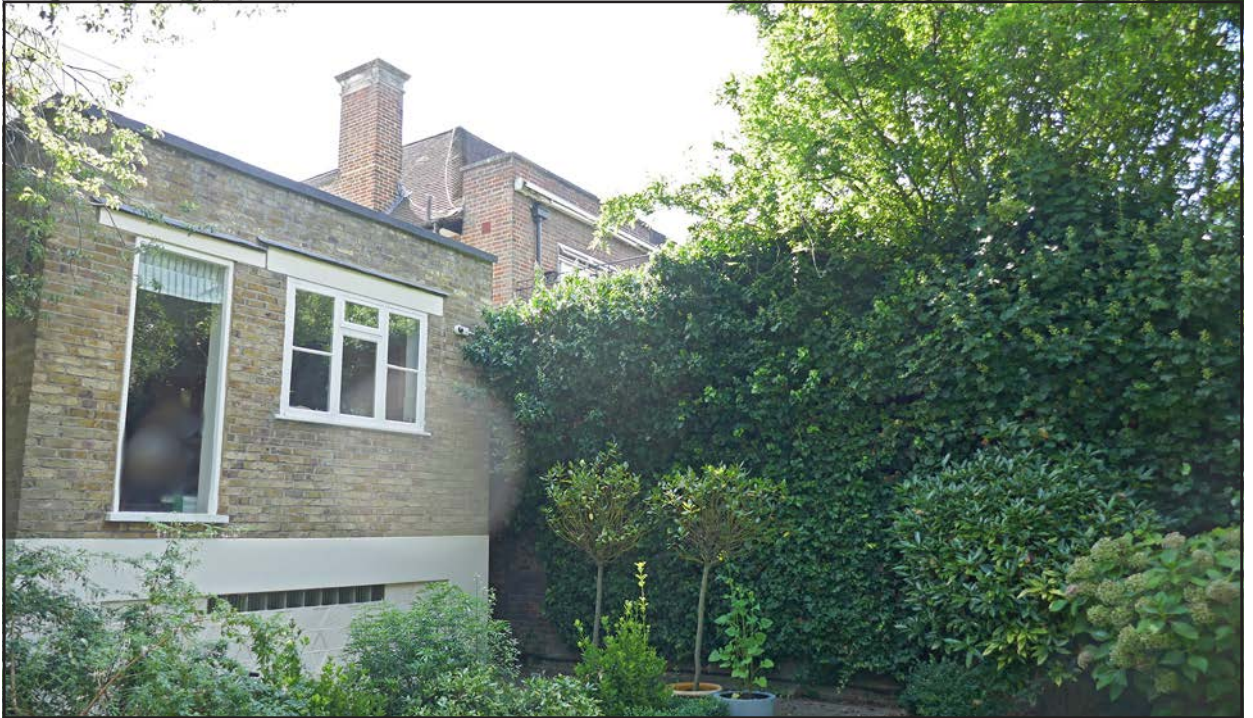
IMG-10 - High site perimeter boundaries
