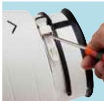
Loosen and open clamps on both sides
