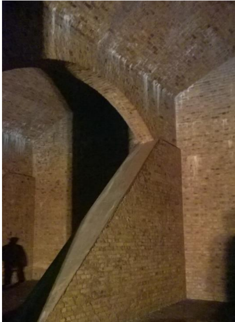
Figure 4: Showing the Existing Masonry Construction
