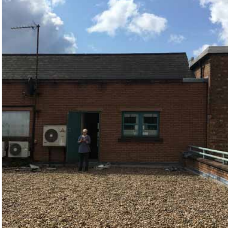
Existing Rear View - Roof Terrace
