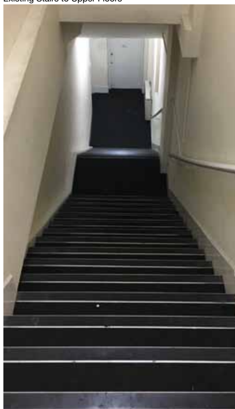
Existing Stairs to Upper Floors
