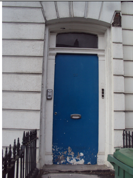
Figure 4 View of Front Door
