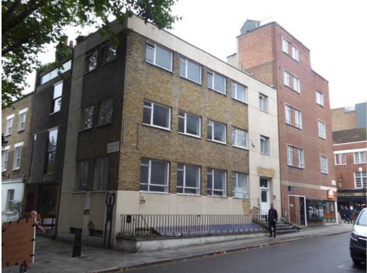
10. View of 27-29 Whitfield Street from east side footway showing abrupt change in height to adjacent building in Goodge Street and obtrusive flank wall.
