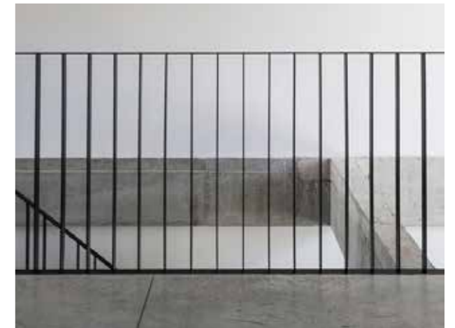
Thin vertical galvanised metal railings are proposed for balustrading as they have low visual impact and an elegant proportion
