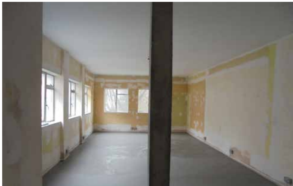
Fig 10: First floor space
