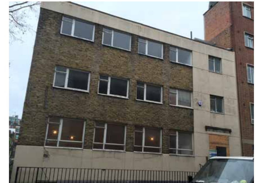
Fig 6 : The existing elevation facing Whitfield Street
