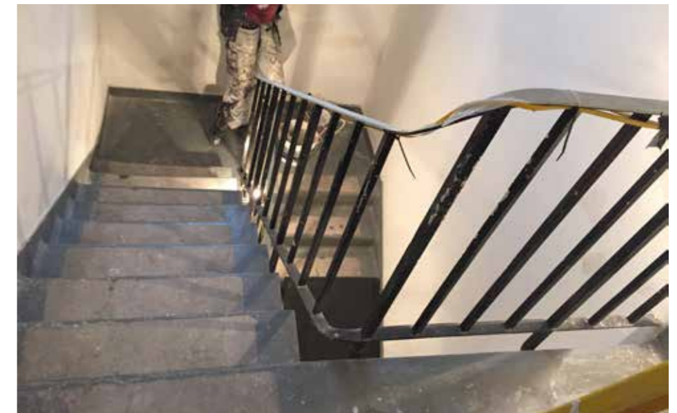
Fig 12: The existing staircase
