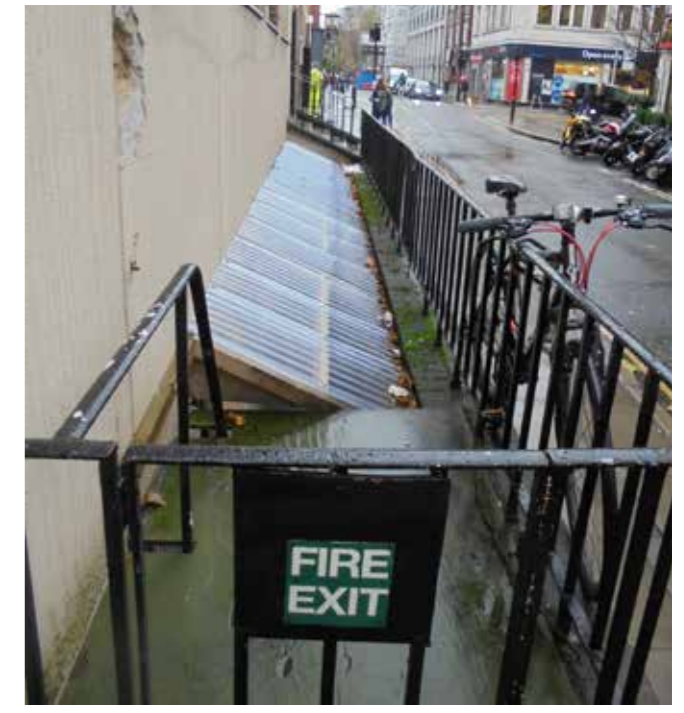
Fig 9: The existing plastic covered lightwell and fire exit
