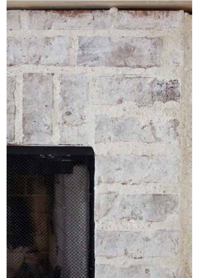
Mortar washed brick wall
