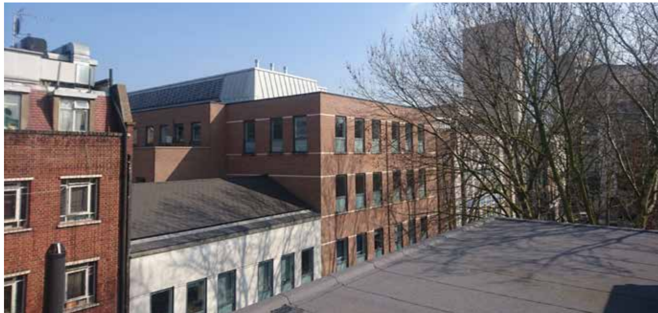
Fig 4 : Rooftop view looking south towards Colville Place
