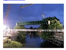
150t sections of a new rail bridge in Lincoln were lifted into place last month by one of the world's largest (1200t) mobile cranes. CGL helped to overcome poor ground conditions with designs to provide temporary ground support for safe operation of the crane under high outrigger and counterweight loads.
