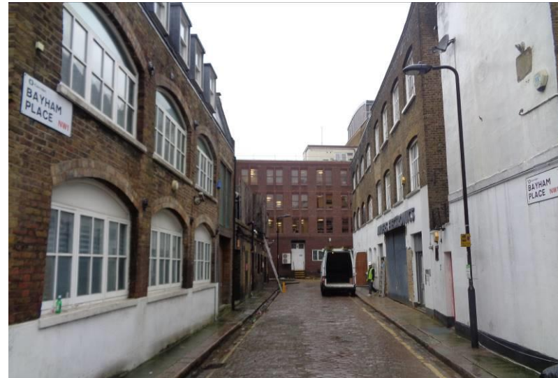
Figure 43: West block of Bayham place looking west.
