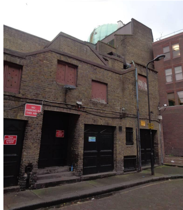
Figure 61: Bayham Place looking south. These mews buildings were substantially altered internally and externally when the theatre was built, though the original facades were retained.
