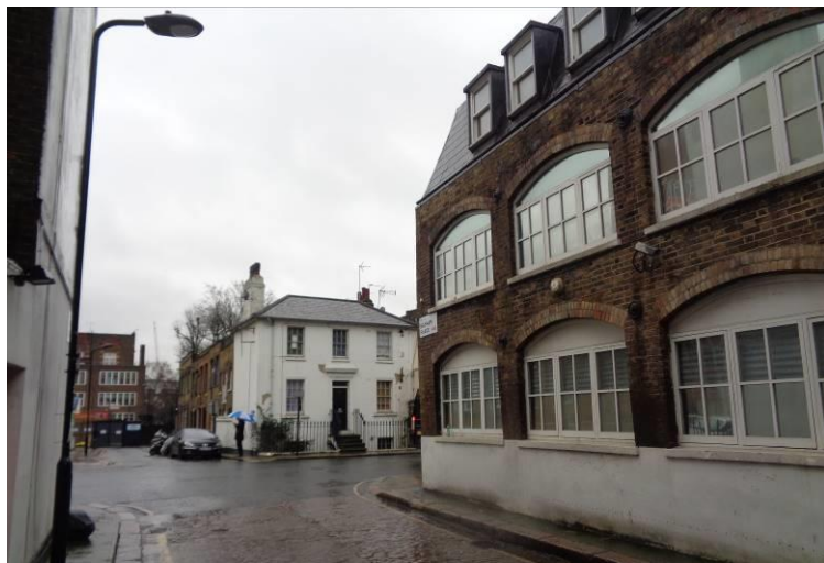
Figure 42: West block of Bayham Place looking east onto Bayham Street. 1 Bayham Place is on the RHS. The major alteration is the roof extension.
