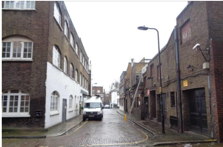
Figure 41: West block of Bayham Place looking east. Mews buildings to the right have undergone alterations to the roofs
