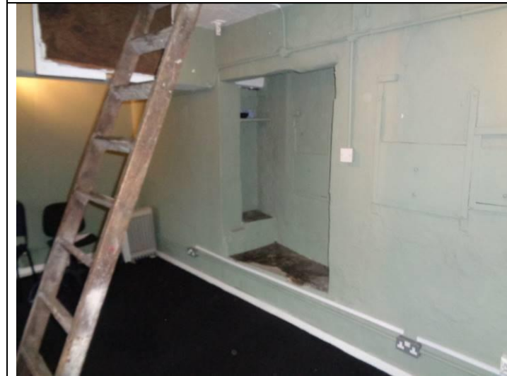
This room was the projection room when the building was a cinema. It sits directly under the dome.
