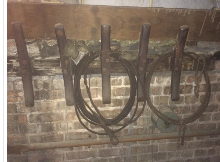
Existing original cleats at fly gallery level
