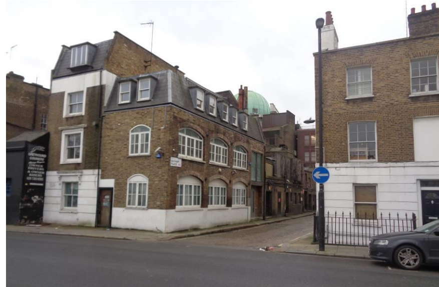
Figure 59: 1 Bayham Street (the narrow building to the LHS) and 65 Bayham Place adjacent (on the RHS). The mansard roofs in both buildings are clearly visible here.
