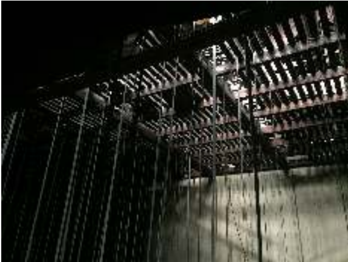
Image 22: View within the flytower looking up through scenographic equipment, lattice and mansard roof.
