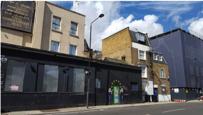
Southern façade of the building
