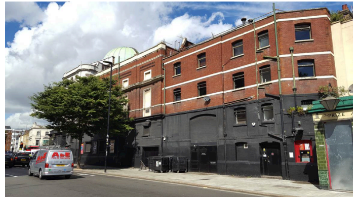
Southern façade of the building
