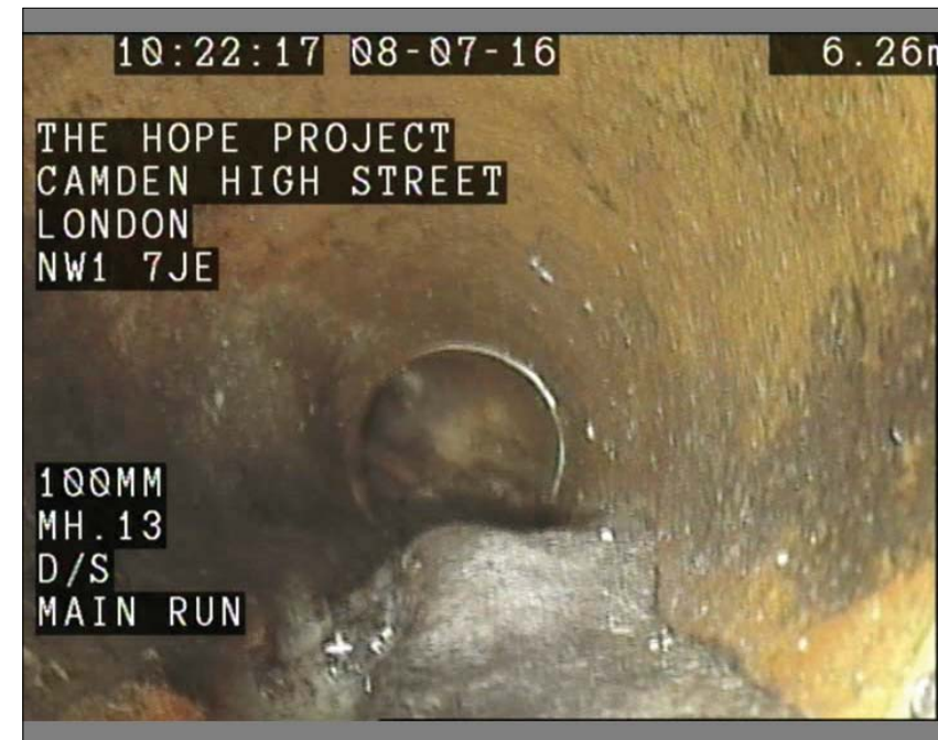
Photo: 33_33_227_A.jpg 6.26m, Attached deposits, encrustation, from 4 to 6 o'clock, 20% cross-sectional area loss
