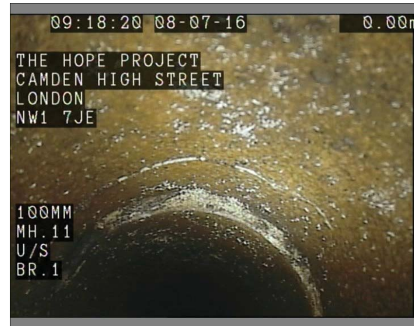
Photo: 25_25_155_A.JPG 0m, Crack, circumferential, from 10 to 2 o'clock
