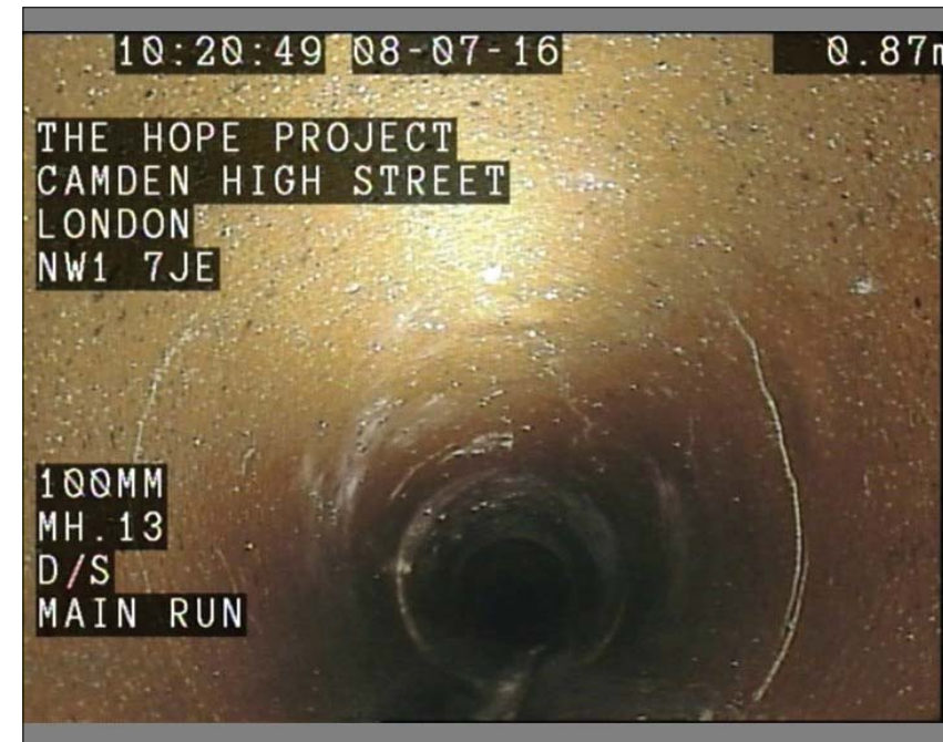
Photo: 33_33_218_A.JPG 0.87m, Crack, circumferential, from 7 to 10 o'clock
