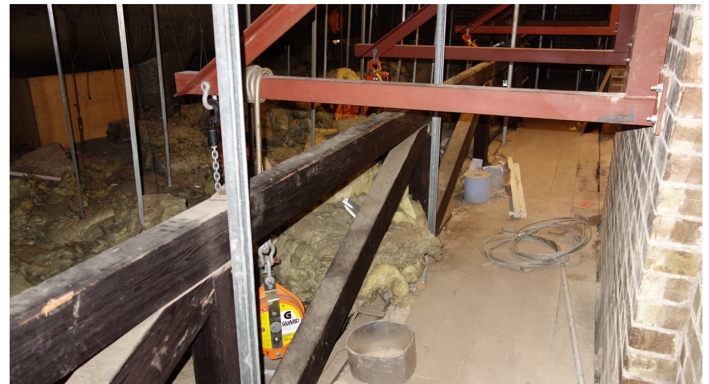
Existing Fly Tower Crossover Gallery Truss
